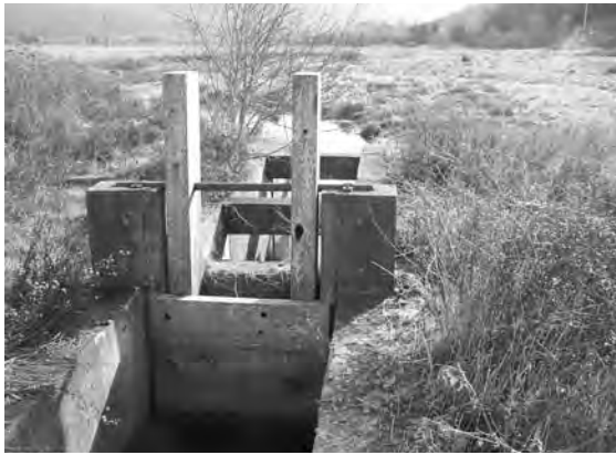
The Freshwater Slough floodgate currently limits flow of water into the wetlands enhancement area.
