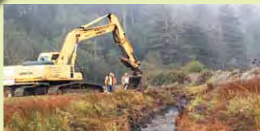
Much effort was made to limit the disturbance of existing wetland vegetation. Disturbed areas will be revegetated, either through the large planting effort scheduled for next spring, or through passive plant colonization.
