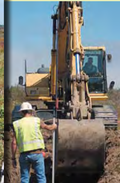
Checking slough channel depth. The project was engineered to facilitate proper sediment transport and drainage throughout the tidal cycle.
