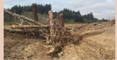
Woody debris installed in Wood Creek as shelter for juvenile salmon
