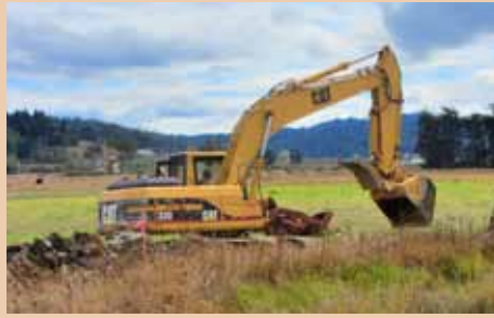
Tide-gate replacement work at Martin Slough
