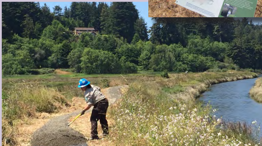
CCC member working on levee portion of trail
