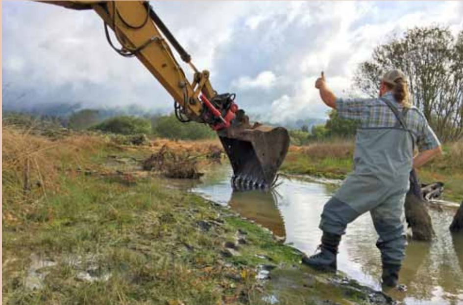
Woody debris installed in Wood Creek as shelter for juvenile salmon
